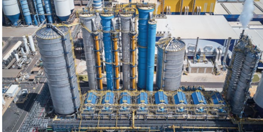
The new hardwood fiberline ensures low operating costs, low emissions, extremely high washing efficiency, and excellent fiber quality. The capacity (6,120 adt/d) is the highest in the world for a single fiberline.
