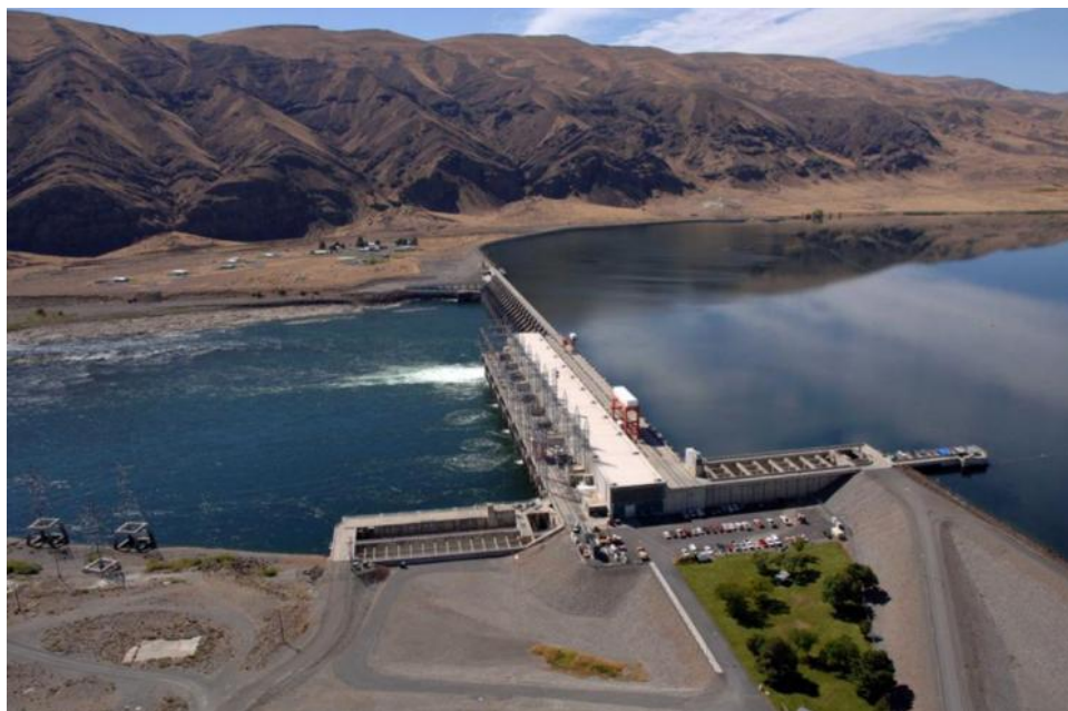
Figure 17 : Priest Rapids Dam
